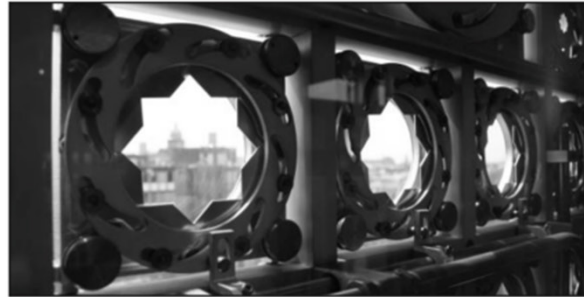
Figure 35: Mechanical system for dynamic screen
